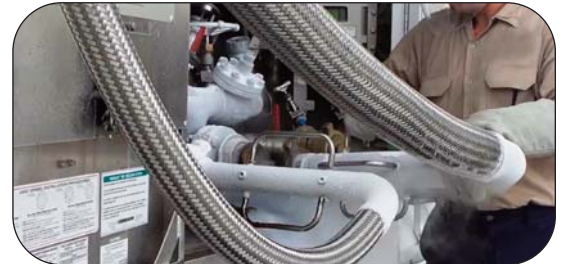
Thorburn HS96Z hose used in a chemical unloading station
