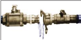
Ordinary Ball Valves Added = Spillage
