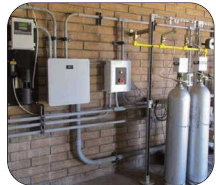
Chlorine gas feed system
