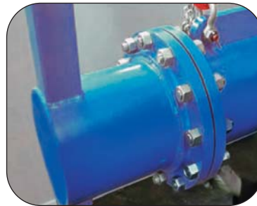
Traditional flanged bolted connection
