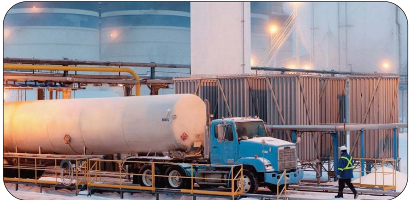
Tanker truck cryogenic bottom loading station
