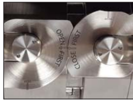
Valve handle locking system
