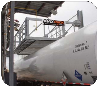
Chlorine gas unloading station
